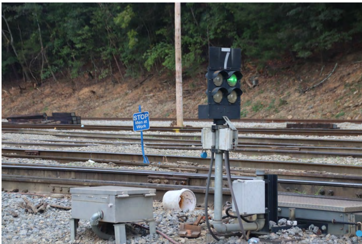
Above and below: Close-up of Wauchatchie Yard air powered switches.
