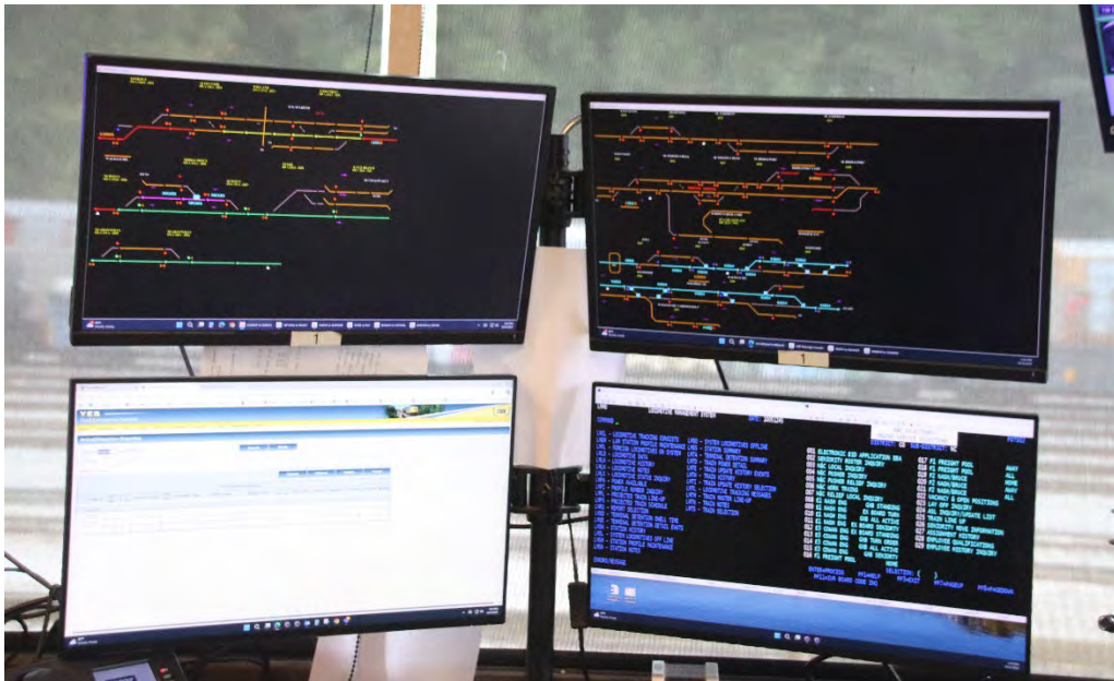
Close-up of the Wauhatchie tower control room track board
