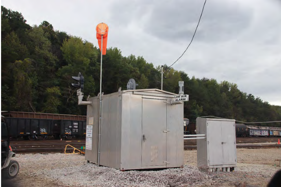
Above and below: The pump house for maintaining air pressure used for remote throwing of yard switches.
