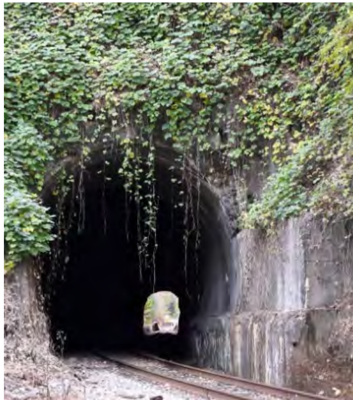
Above and next page: R240-02 heads back west toward Shelby and is approaching the tunnel at Douglas.
