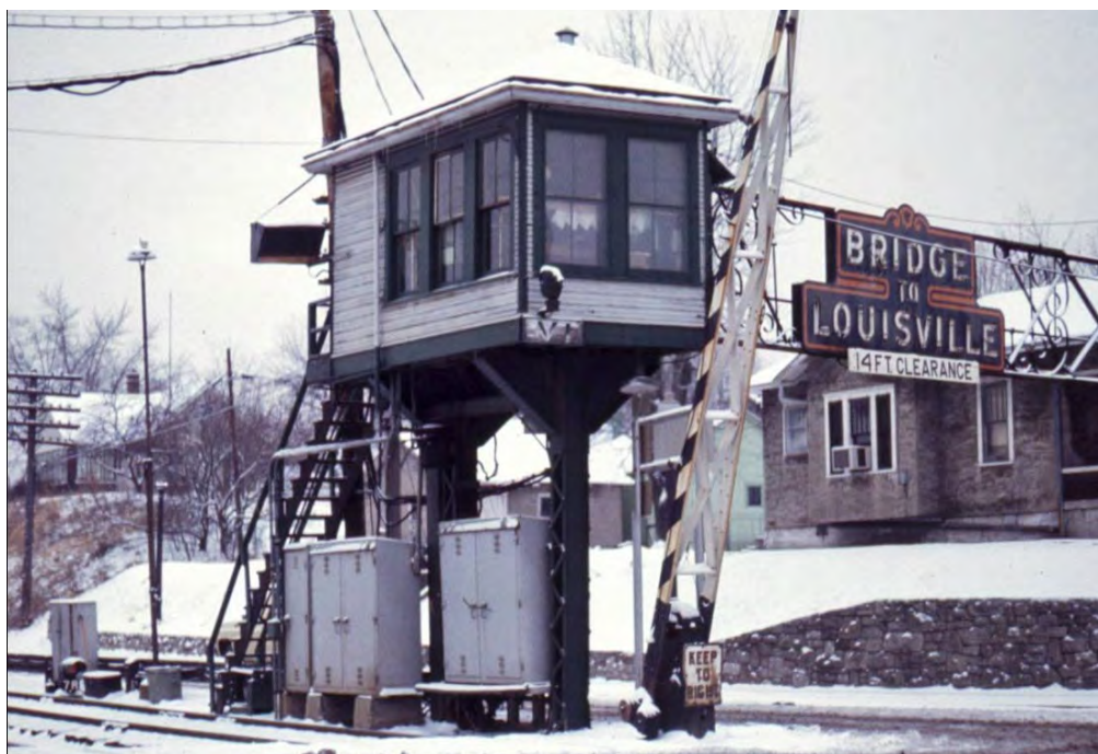
A closeup of VI Tower controlling entrance to the north end of the K&IT Bridge. (University of Louisville Archives)
