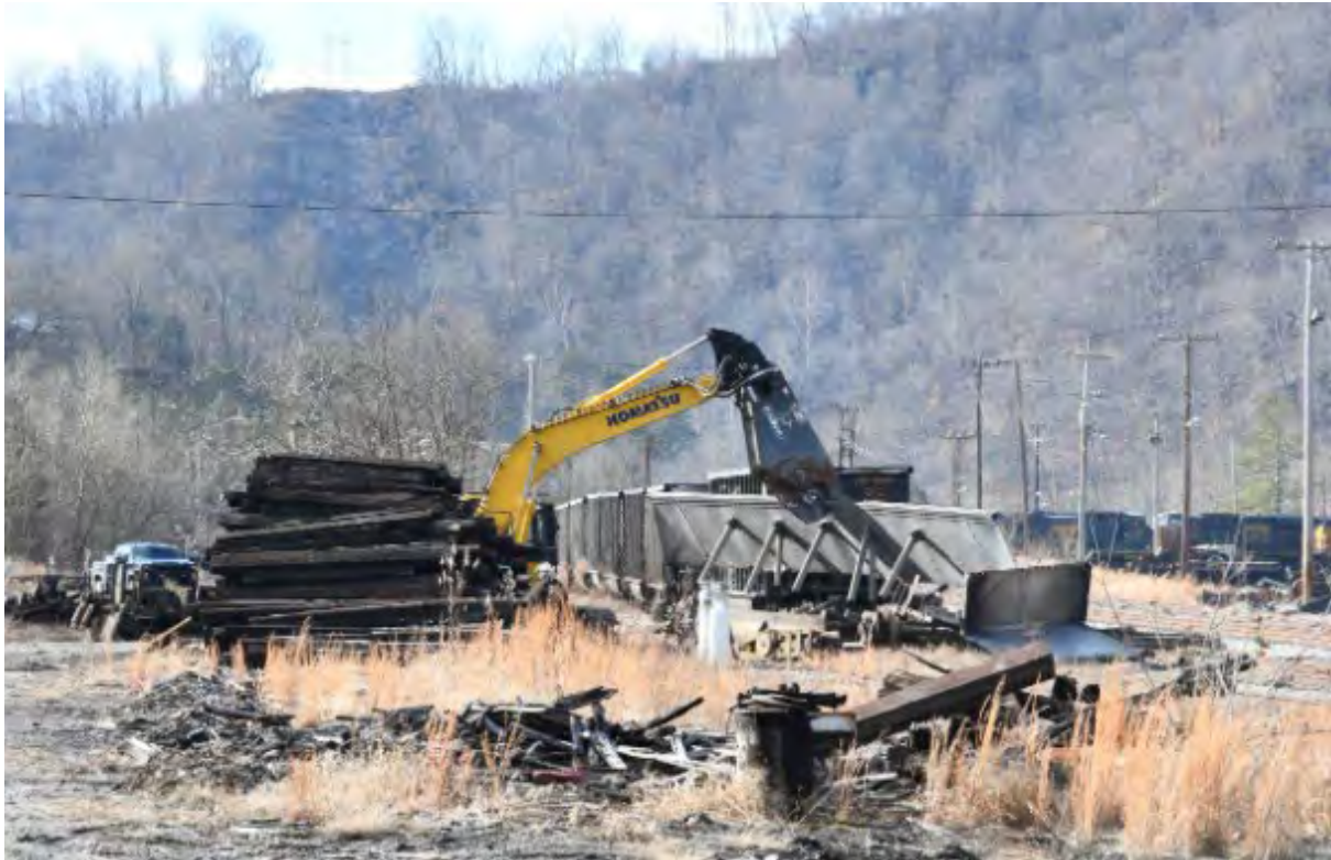
This page and top of next page: Some of the tubs from Esco were repaired, but others were scrapped at Shelby. 1-19-26
