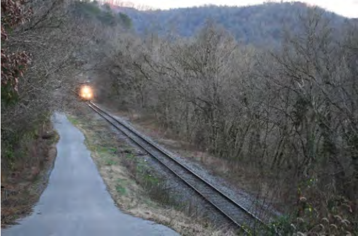
Crossing the county road at Hite, Kentucky, MP 1 from Martin Jct.
