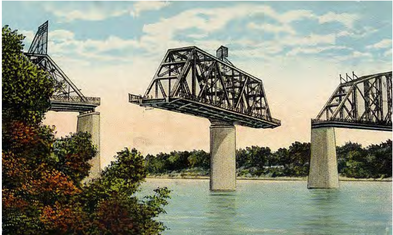
The swing span being tested
