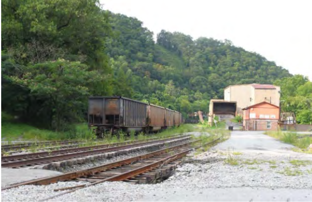
The tracks were flooded by Shelby Creek at Esco, Kentucky to a level above the trucks on the coal tubs.
