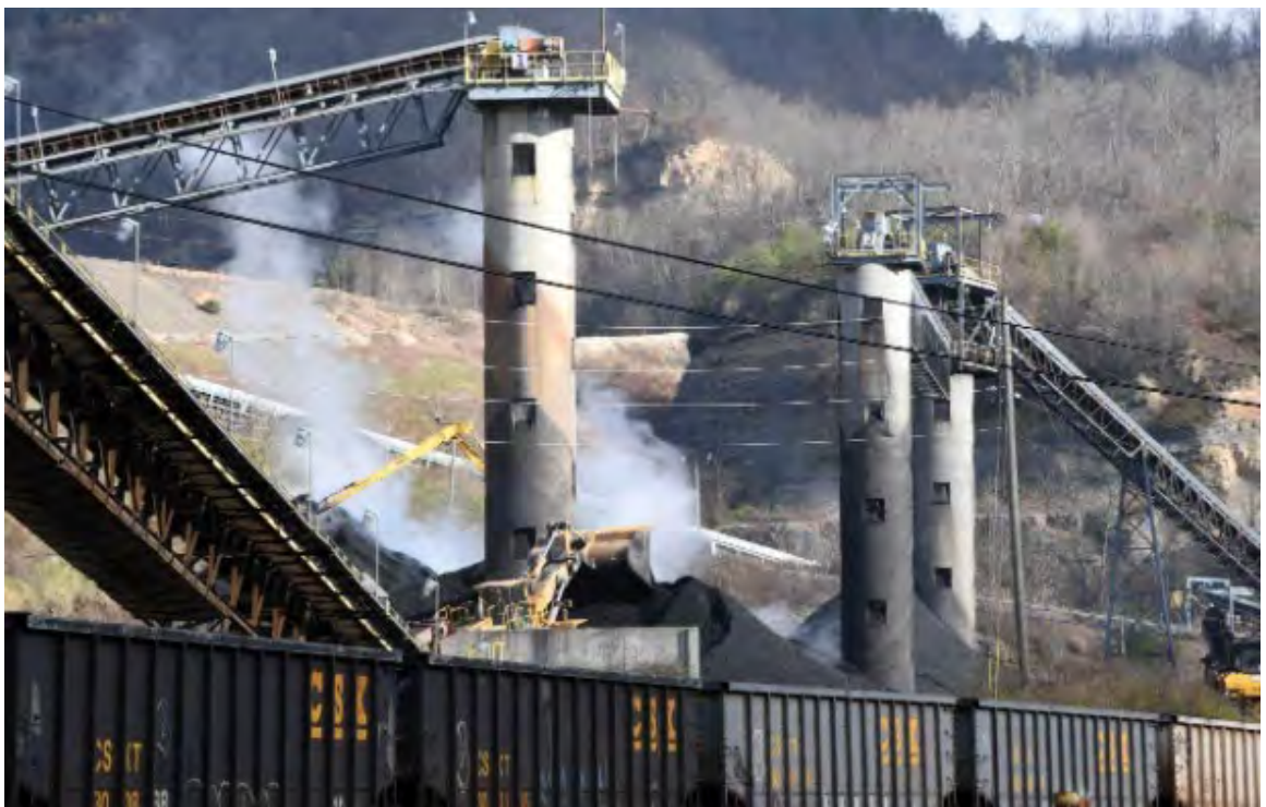
A dozer keeps the stockpile heaped up.
