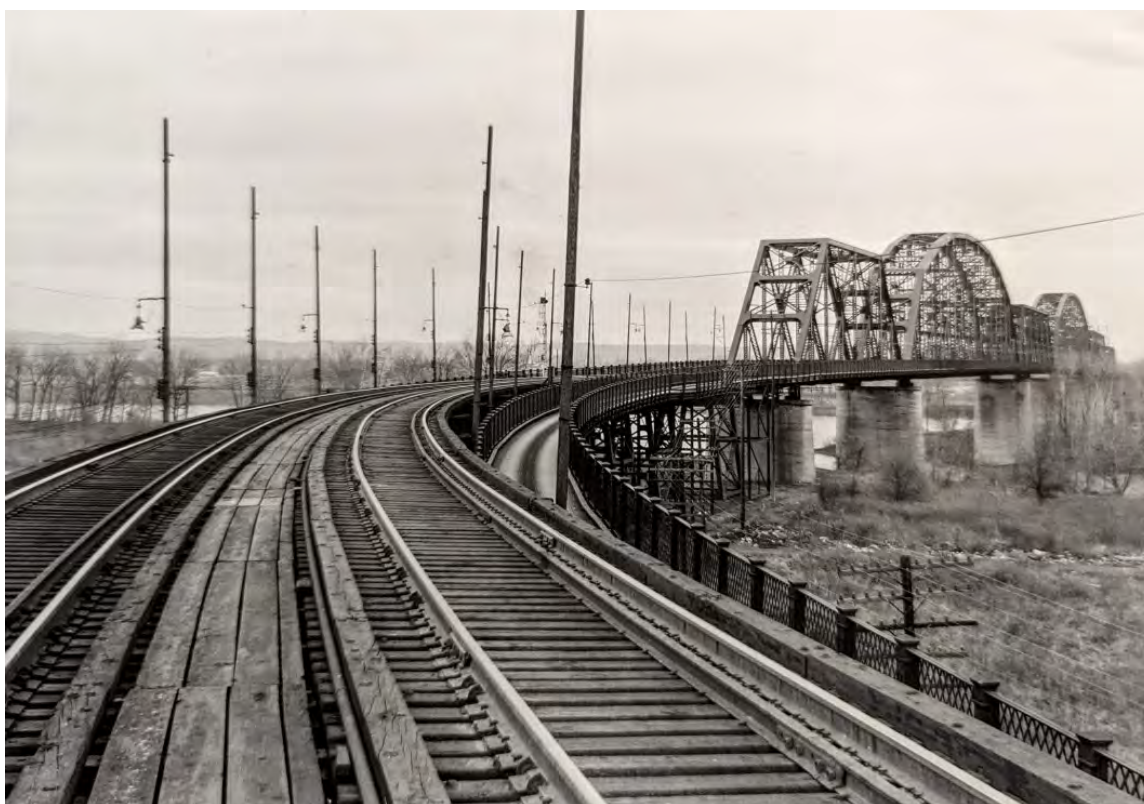
View of K&IT Bridge from Kentucky shore. (University of Louisville Archives)
