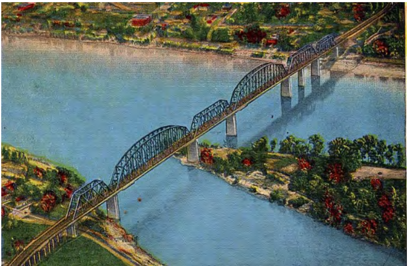
The K&IT Bridge from the Kentucky shore to the Indiana side. Waterway in bottom of photo is downriver entrance to the Portland Canal. Second span in from Indiana shore is swing bridge
