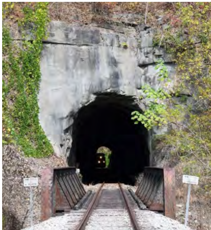
Above and next page: The SV&E circumvents a big bend in Shelby Creek by utilizing this 744' tunnel between Robinson Creek and Douglas, Kentucky. It was damaged by arson in 2015 and underwent extensive repairs. We're on the Douglas end at around MP 6. This tunnel was excavated in 1912.
