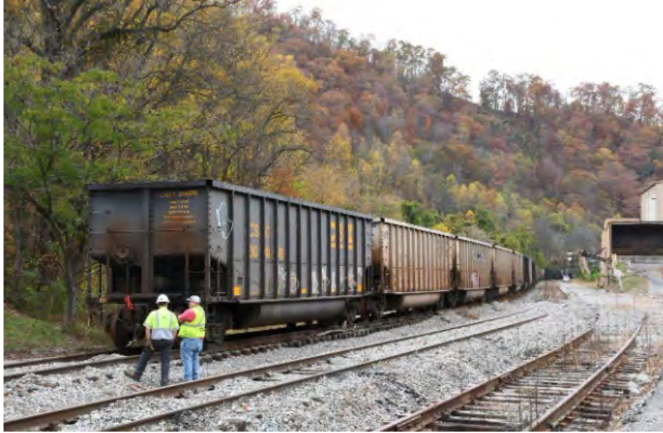
Attaching the red flag and visually inspecting the tubs before moving. CSXT MofW has filled the washouts with ballast.
