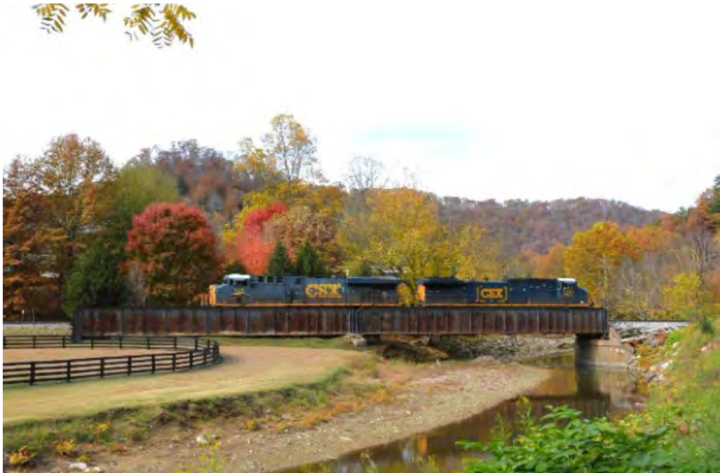
Another half mile, R240 crosses Shelby Creek again at Yeager. Kentucky.
