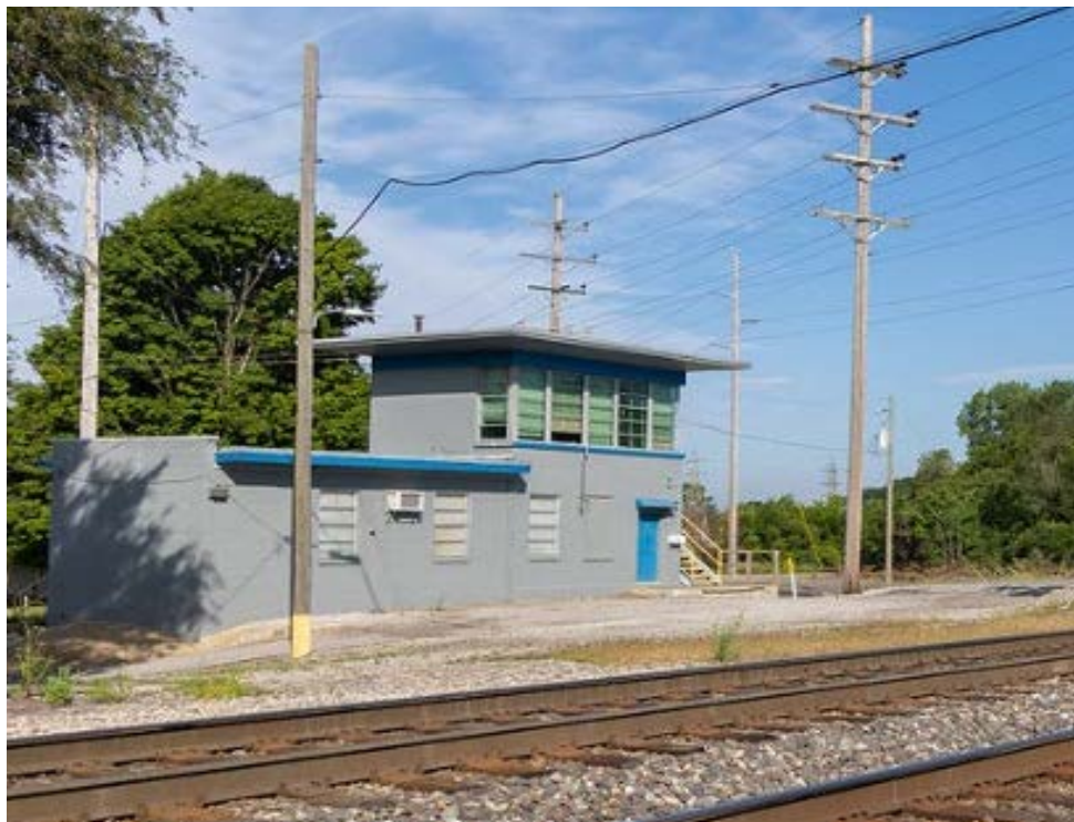
Left and trackside view of building
