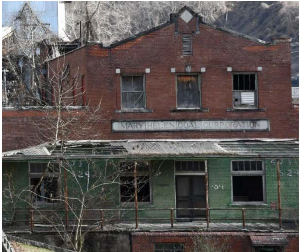
One of the last old company store buildings left in the Southern Appalachians. It could be demolished at any time.
