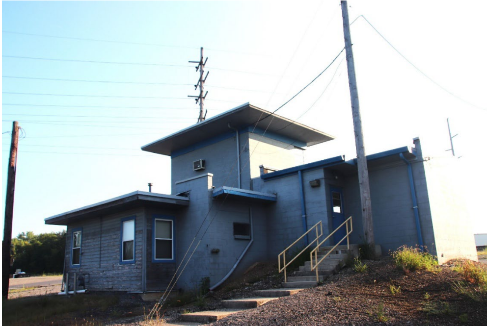
Back and left side of building
