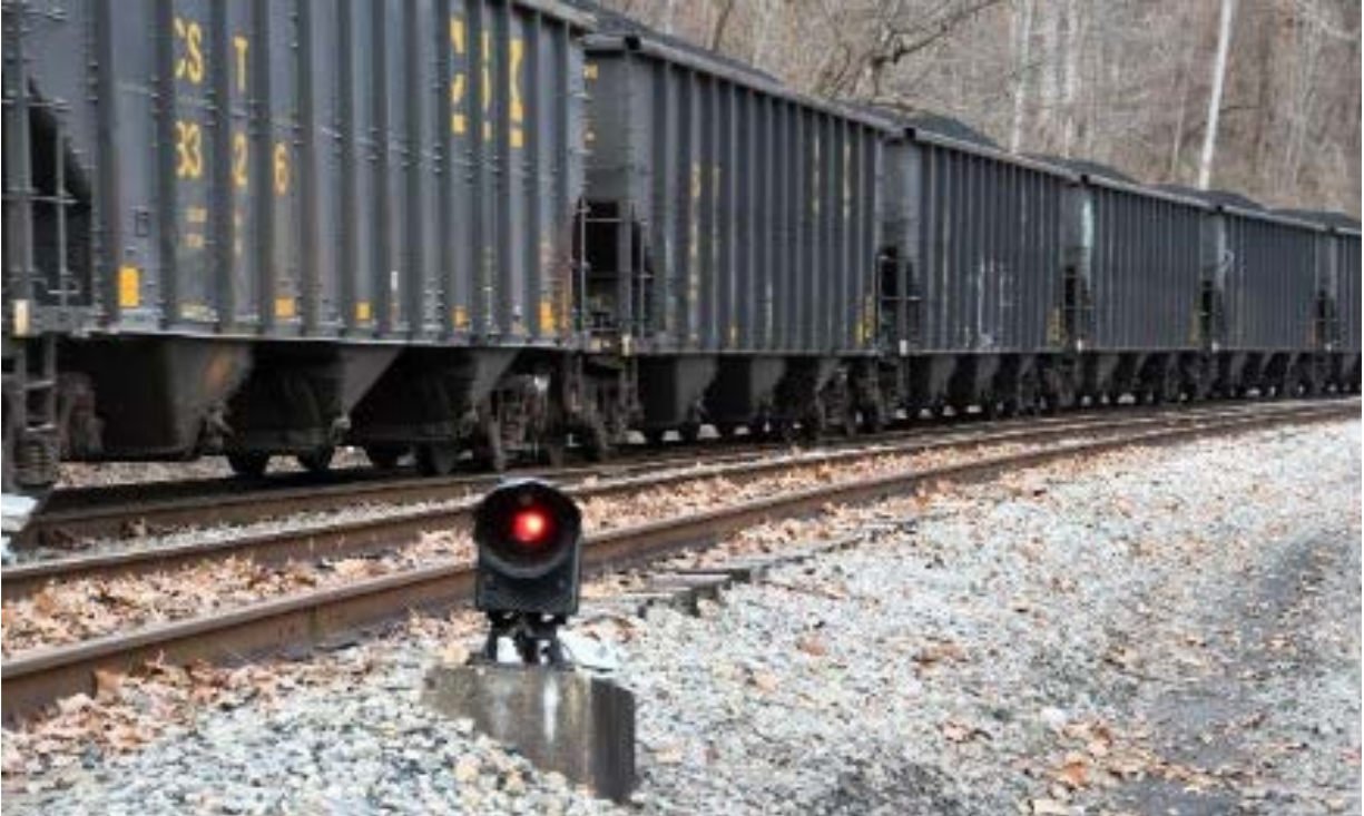
Dwarf signal on the controlled siding at North Loyall looking south.
