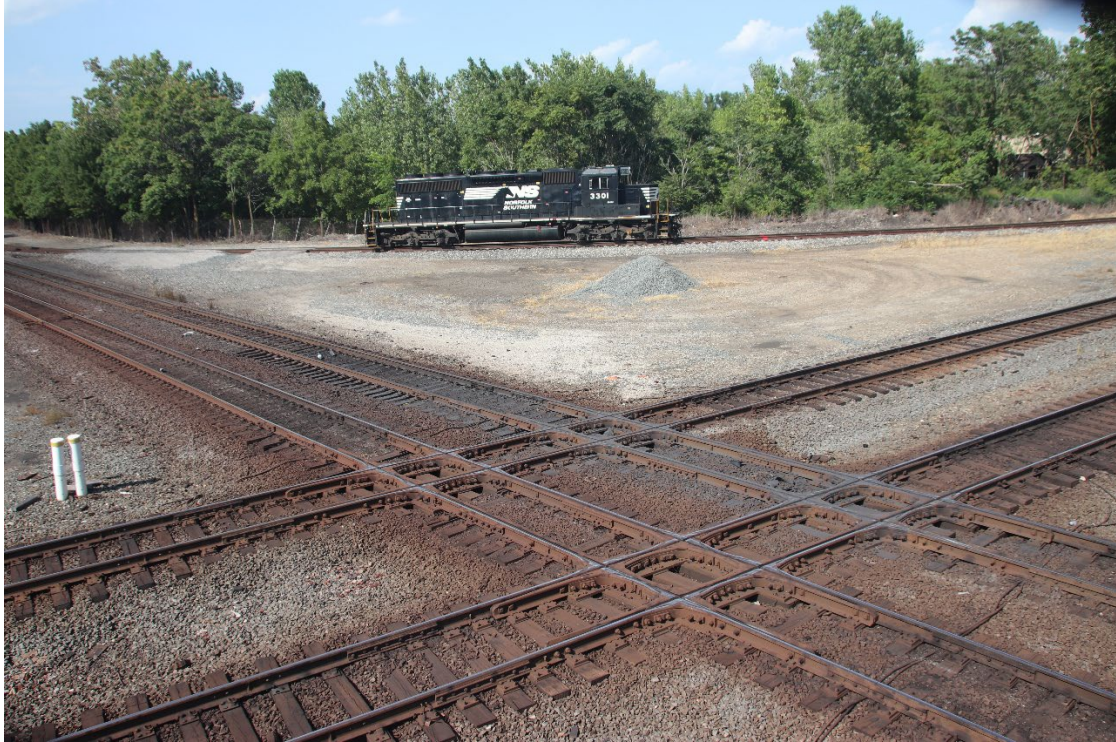
One of the two diamonds at the Marion Depot. From top left to bottom right is Norfolk Southern track and from top right to bottom left is CSXT track.
