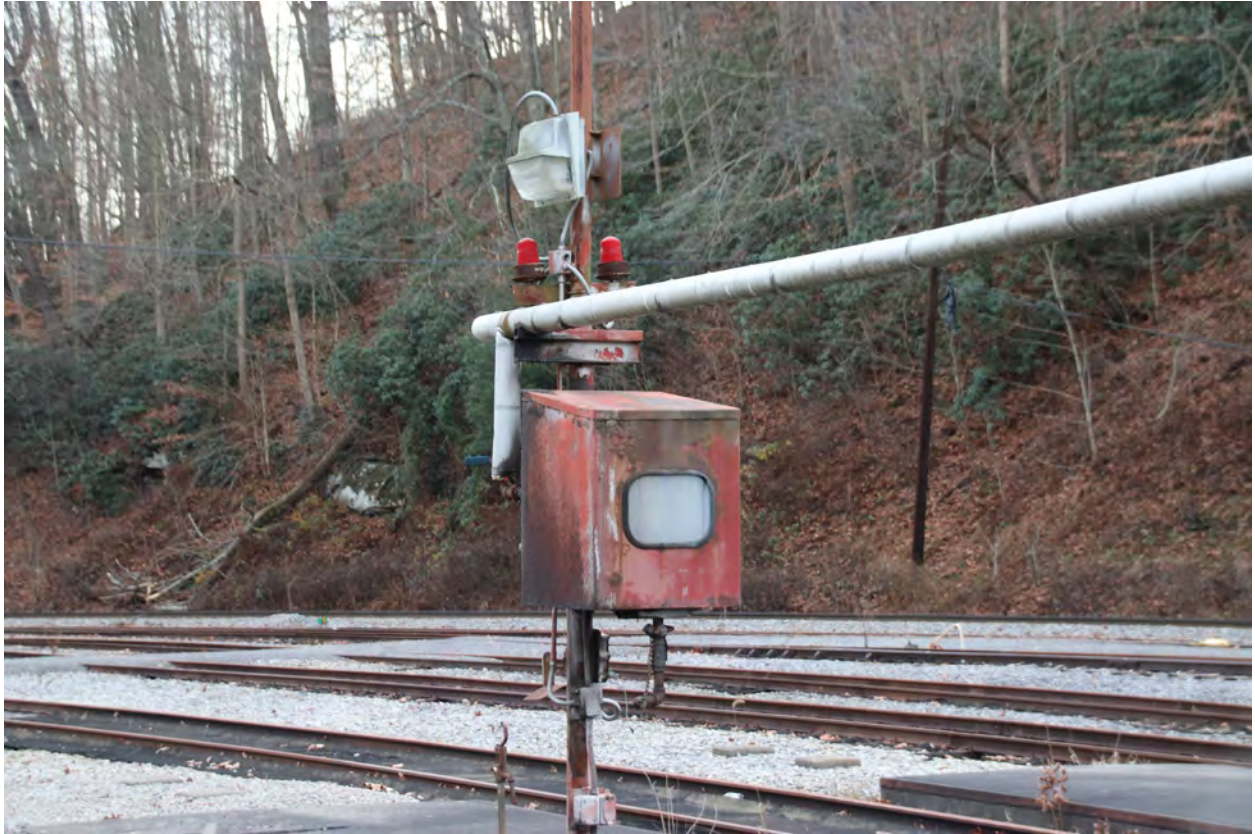
Close-up of the south end of the refueling pad
