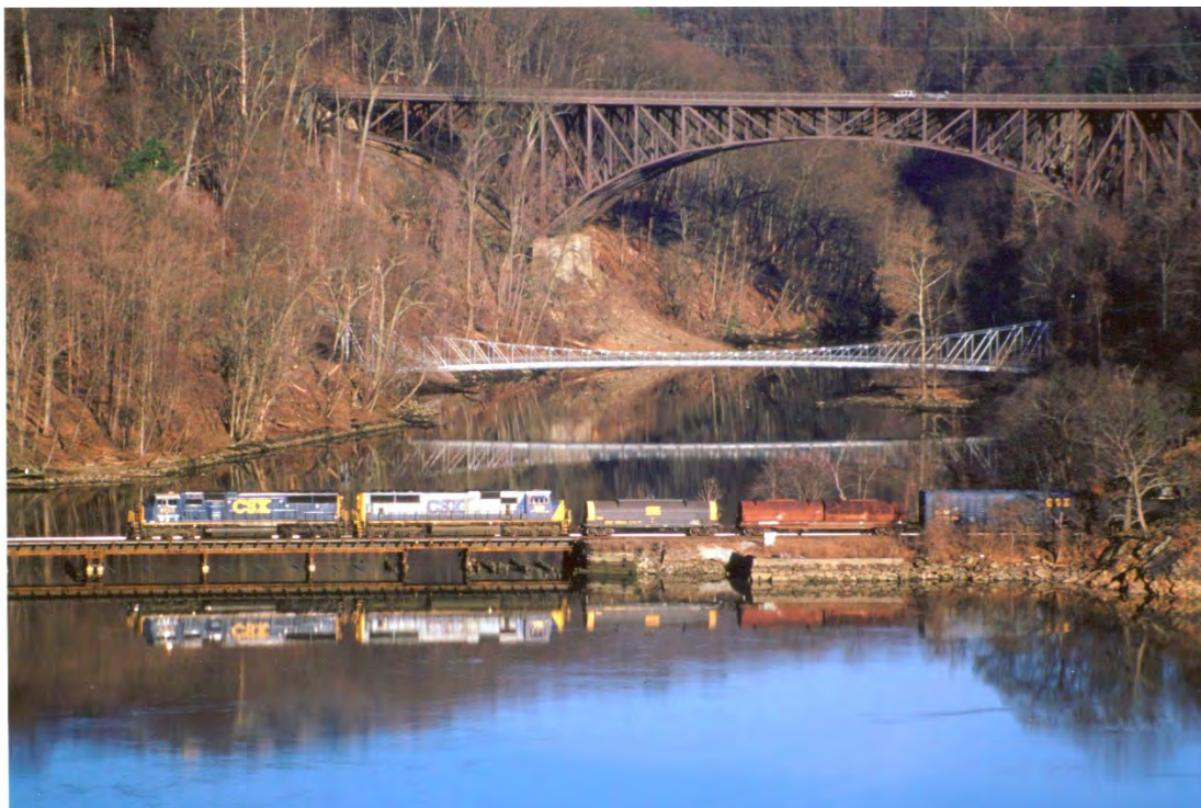
Two CSXT locomotives are seen here crossing the bridge over Popolopen Creek, Mile Post QR 42.5, as they head down the Hudson River for New York City. The train is just exiting the Fort Montgomery Tunnel. In the background is the Popolopen Suspension Bridge. (Richard Herbert)
