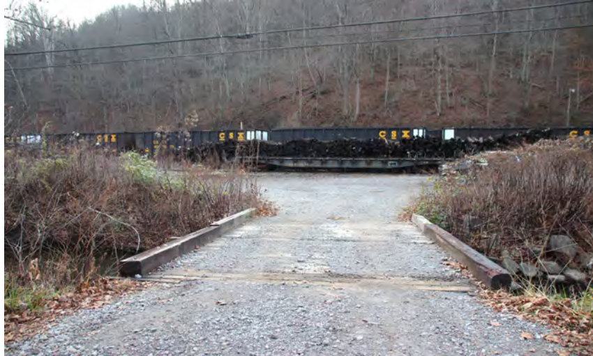
The bridge leading off Virginia 83 into the southern end of CSXT's Dante Rail Yard
