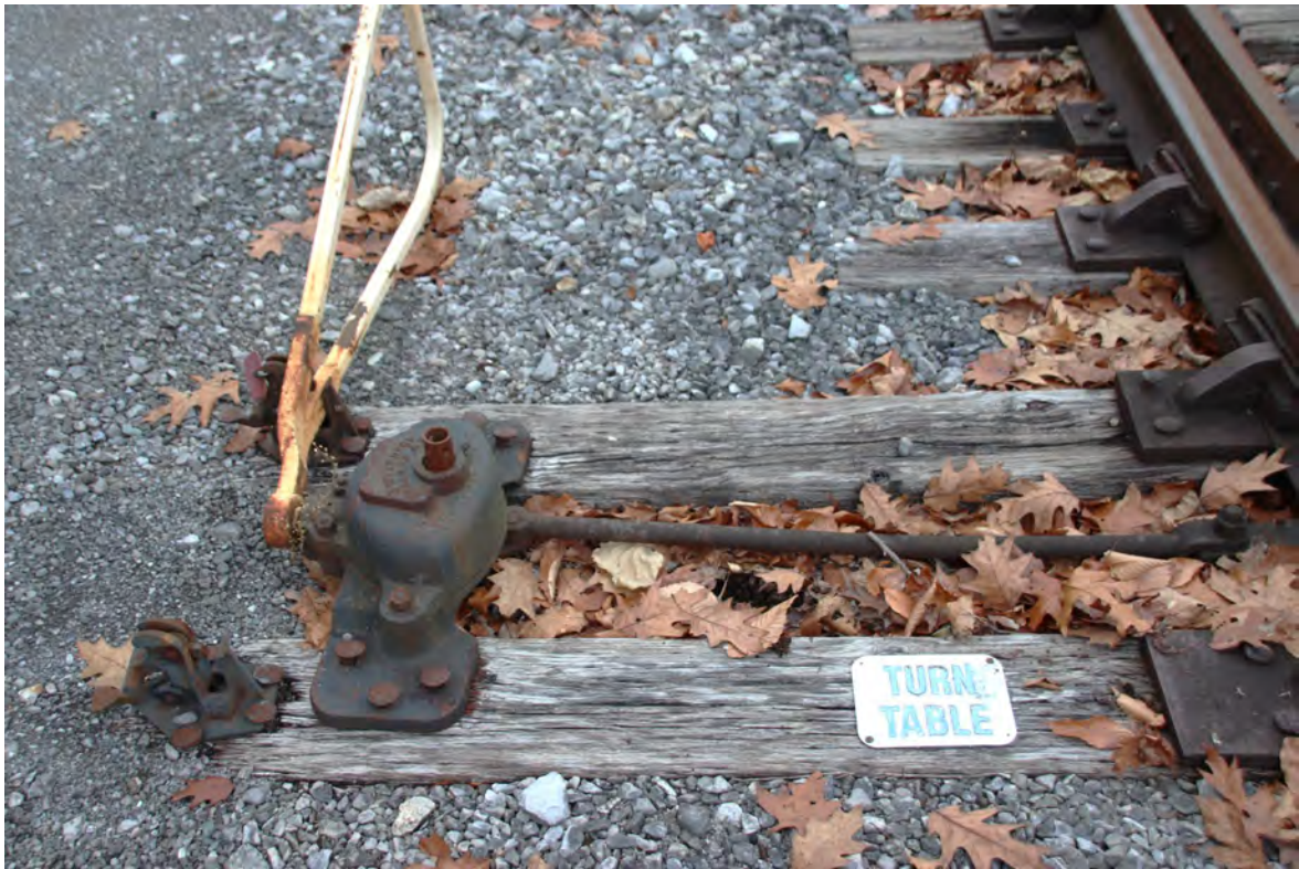
Switch from the mainline to the turntable.
