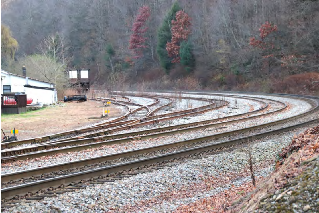
Entry track into the Receiving Yard
