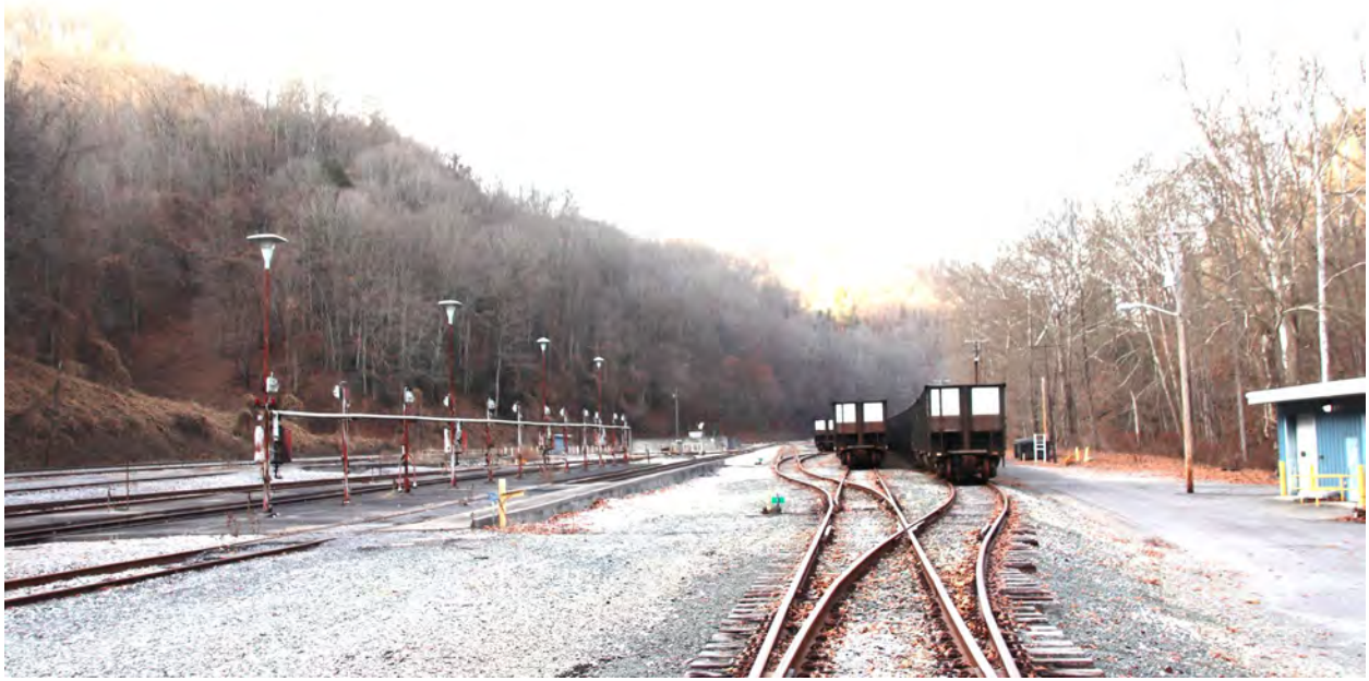
The Service Yard. The yard office is on the right, the fuel pad to the left, the turntable just beyond.
