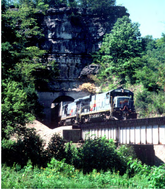
A CSXT train with Seaboard System locomotives is seen running south on the KC Line between Cincinnati, Ohio, and Corbin, Kentucky, in August of 1986. Led by CSXT 5877, the train is southbound for Corbin. She is seen exiting Tunnel 15, the “Eye of the Needle,” and crossing Brush Creek. (Richard Herbert)
