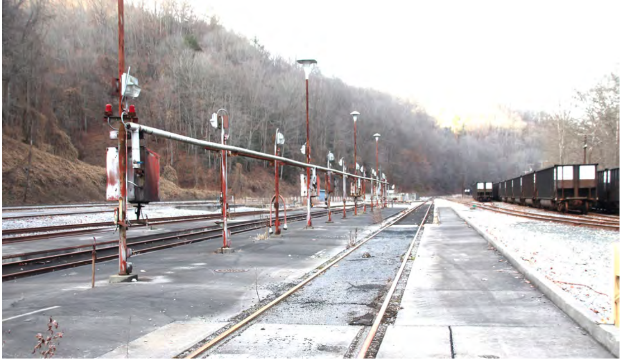
A view north from the south end of the abandoned fuel pad
